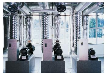
Bolier flow rates controlled by variable speed pumps
