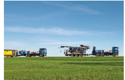
Ground drilling with BauGrund Süd
