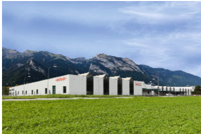
Heating system production Facility in Sennwald, Switzerland
