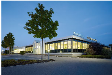
Neuberger Building automation in Rothenburg o.d.T.
