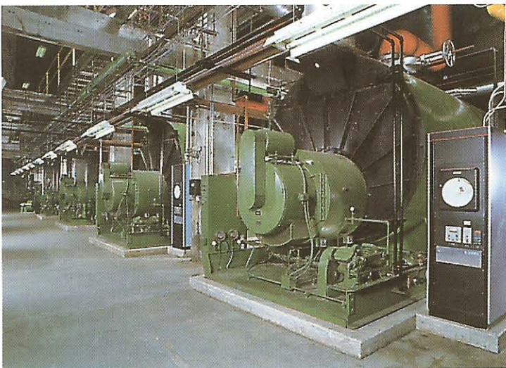
Merchandise Mart – Chicago, IL (2) 750 HP, (1) 500 HP, (1) 150 HP Gas/Oil Burners, Low Pressure Steam
